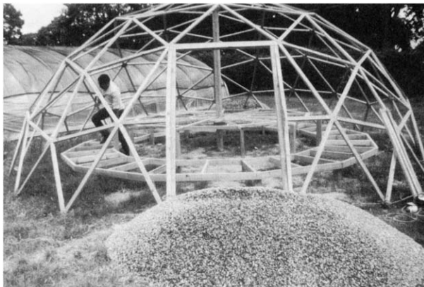
FIGURE 11 Structure of geodesic dome dryer.
